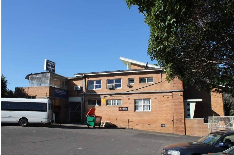
Figure 7 – Side view of ex-Club building and at-grade car park
