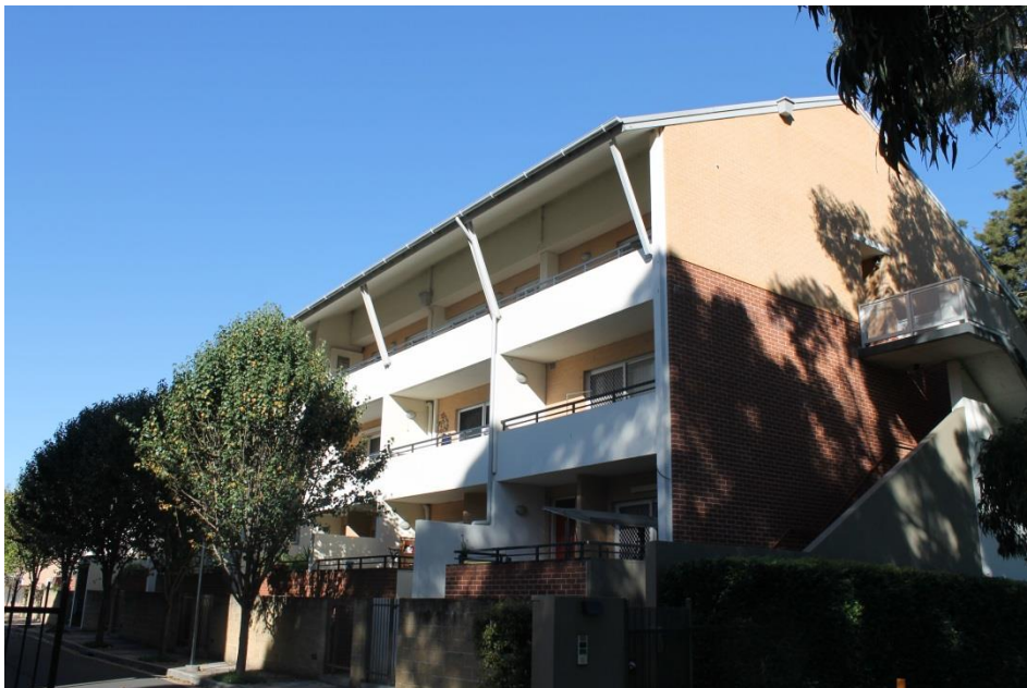
Figure 11 – The Sugar Mill development at the site's eastern boundary
